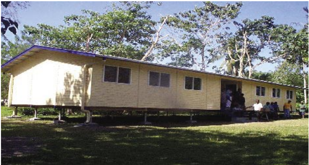
Double classroom at Koimumu Primary School, Hoskins.
